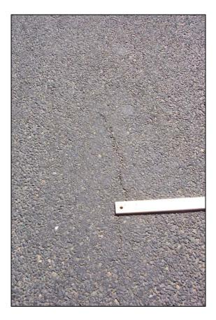
FIGURE 9: Low Severity Longitudinal Cracking
