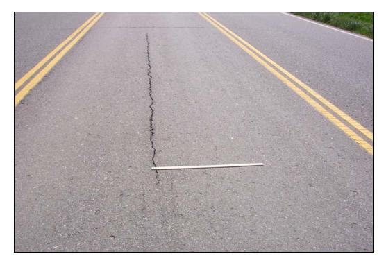
FIGURE 8: Medium Severity Longitudinal Cracking
