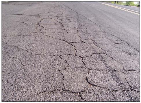
FIGURE 5: Medium Severity Alligator Cracking
