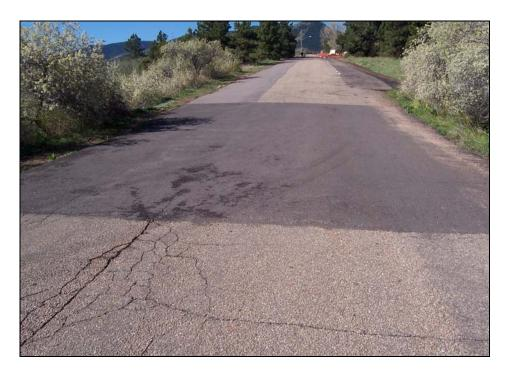
FIGURE 17: Full and Partial-Width Road Patching
