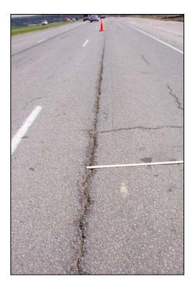
FIGURE 7: High Severity Longitudinal Cracking
