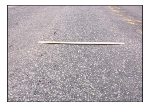
FIGURE 20: Medium Severity Rutting
