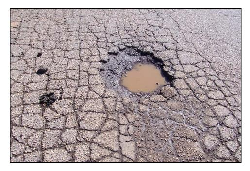
FIGURE 16: Pothole Surrounded by Alligator Cracking
