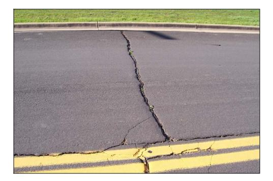
FIGURE 10: High Severity Transverse Cracking
