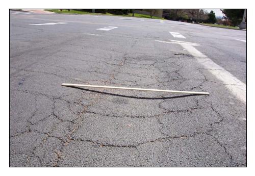
FIGURE 19: High Severity Rutting
