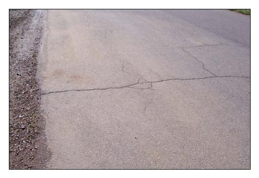
FIGURE 11: Medium Severity Transverse Cracking
