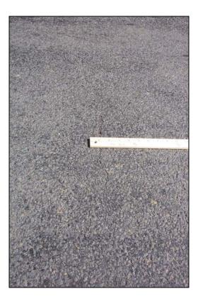
FIGURE 12: Low Severity Transverse Cracking
