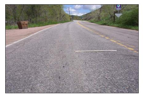
FIGURE 21: Low Severity Rutting
