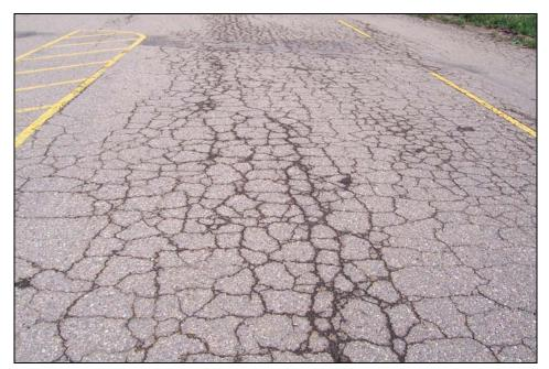
FIGURE 4: High Severity Alligator Cracking
