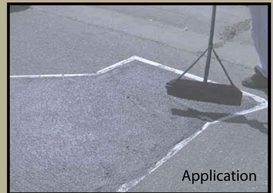
GatorGuard Protects the sub-base by forming a durable, water-tight covering.
